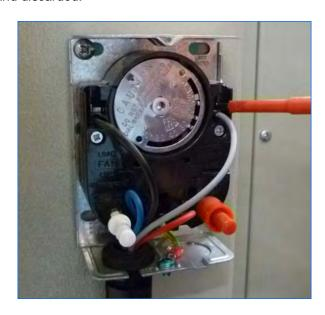
Unscrew and withdraw cable gland (save for later), then remove fixing screws then remove unit from heater.
