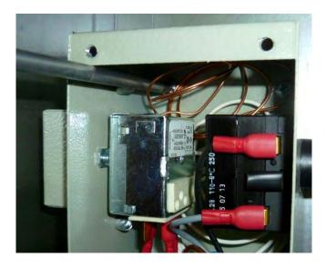
Fit the supplied female spade crimps to the original cables .
